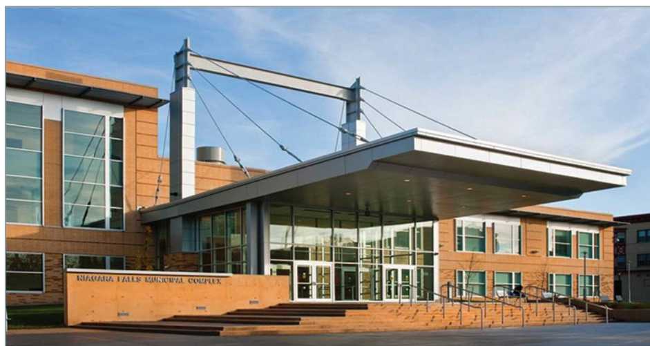
Niagara Falls Police State and court complex. This modern complex was built in 2009 for $40 million and houses 4 courtrooms, the city jail, and police headquarters.
