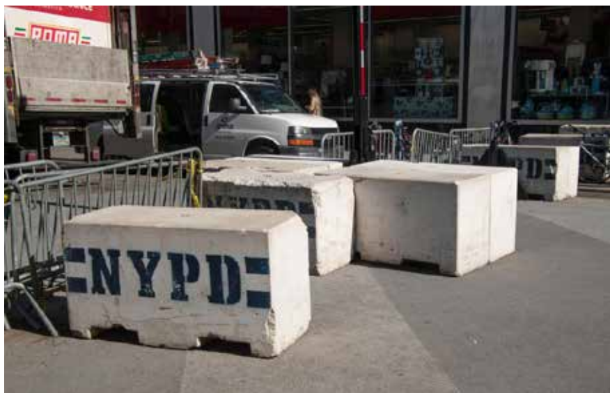
Countermeasures that would be deployed to prevent a VBIED attack, such as bollards, jersey barriers and heavy blocking vehicles would also hinder someone bent on a vehicle ramming attack.
